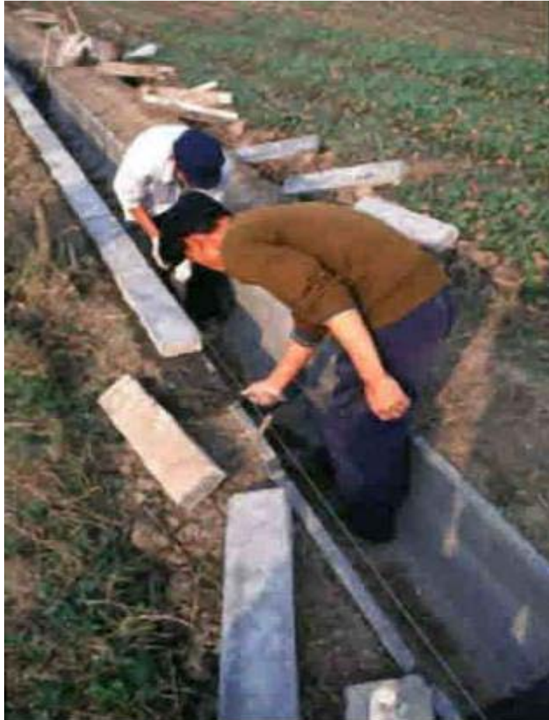
Plate 12 : Construction of concrete irrigation ditches will prevent breeding of Oncomelania snails (Source: WHO/TDR/ Crump)
